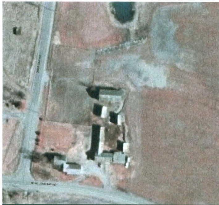
2003 Color infra-red image of a portion of the Lewis Farm where the farm employee housing was constructed. These structures were demolished prior to building the employee housing cluster.
