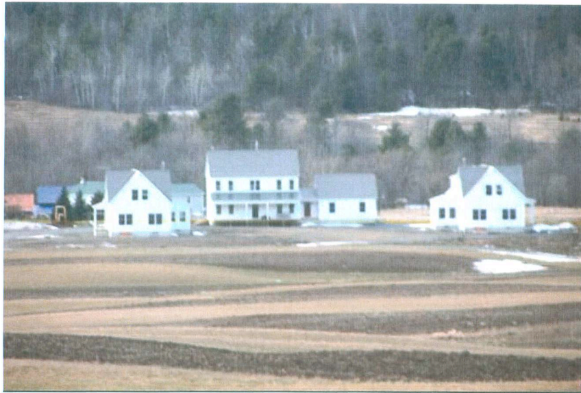
This is a 2008 image of the clustered housing on the Lewis Family Farm. Homes will be used to house farm employees. The housing was constructed on the same footprint where a home and barns existed in the 2003 image. The edge of the Hamlet of Whallonsburg, no more than 200 feet away, is evident behind the South Family Cottage.
