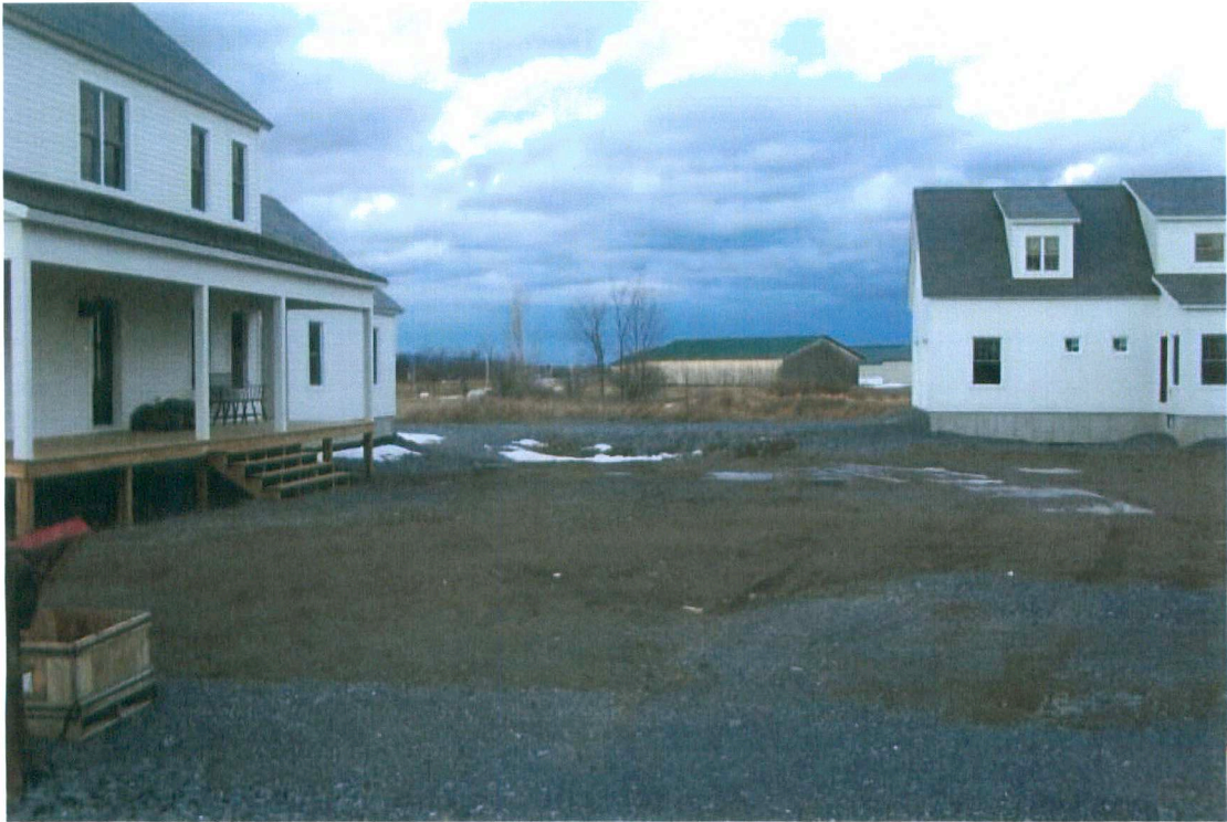
Barns housing the farm's equipment is located adjacent to the clustered homes. Common yard will contain the leach field, which will be used by all three of the homes.
