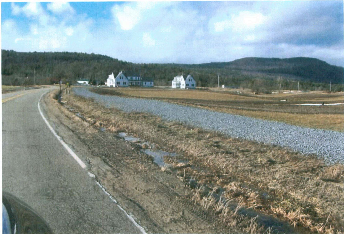
Farm employee housing clustered together with a combined leach field that will be used by all three structures. The Homes are located in close proximity to the barns.
